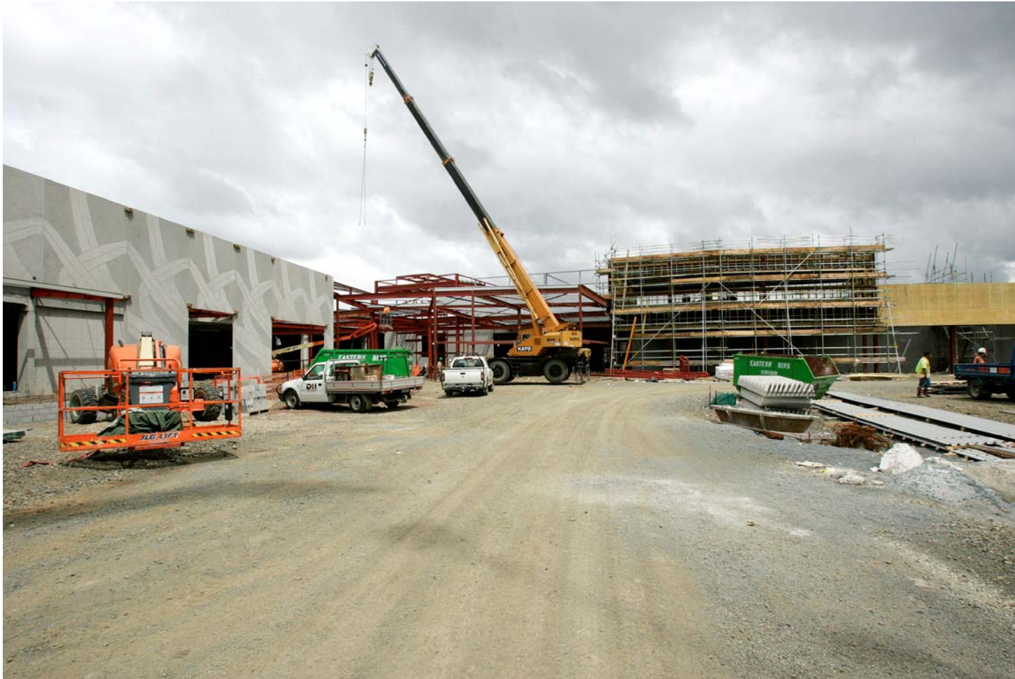
Exterior of Main Entry – Stage 1
