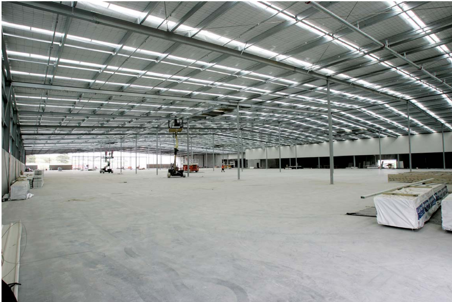
Interior of the Warehouse – Stage 1
