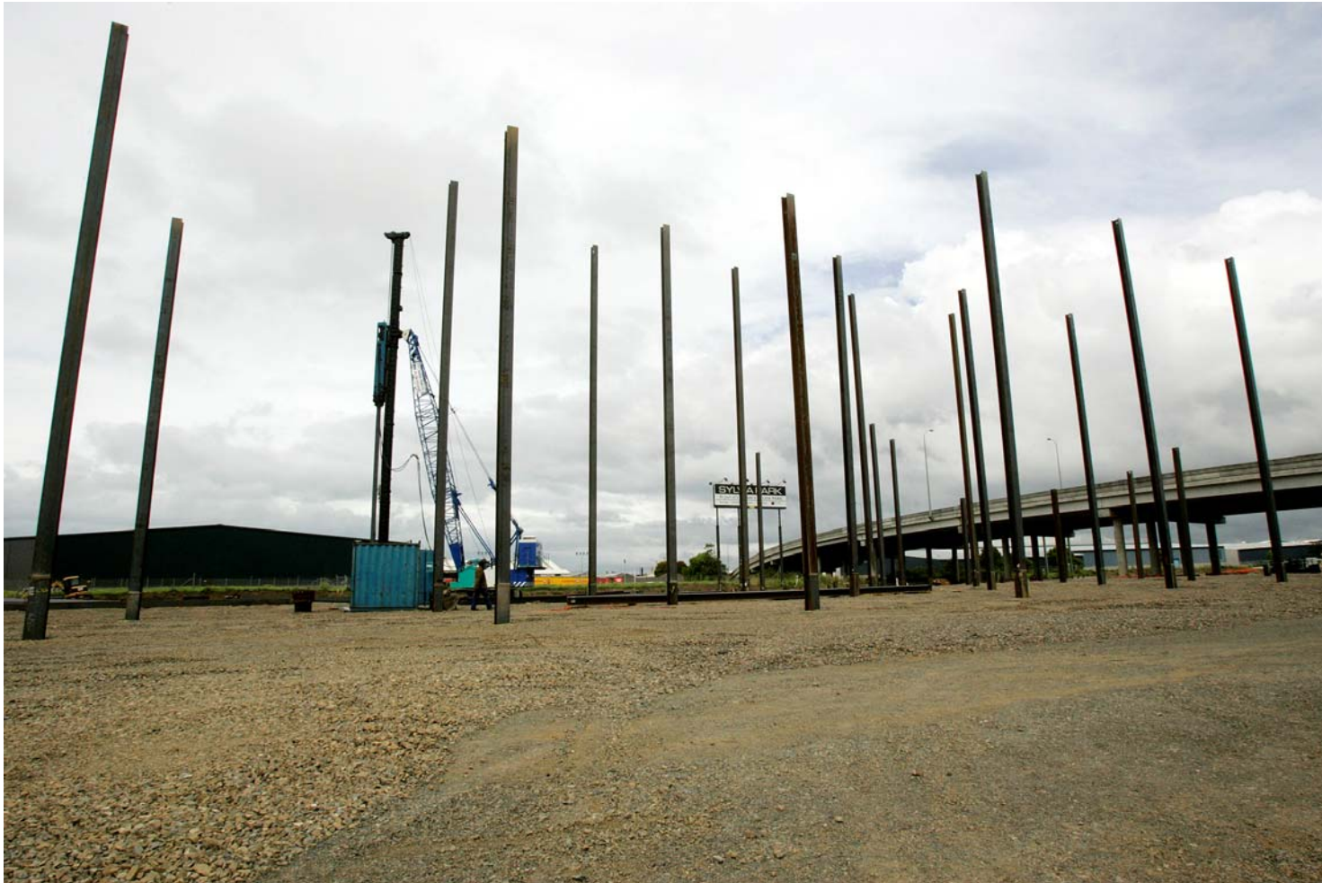
Piling for the ELP Cinema precinct – Stage 3
