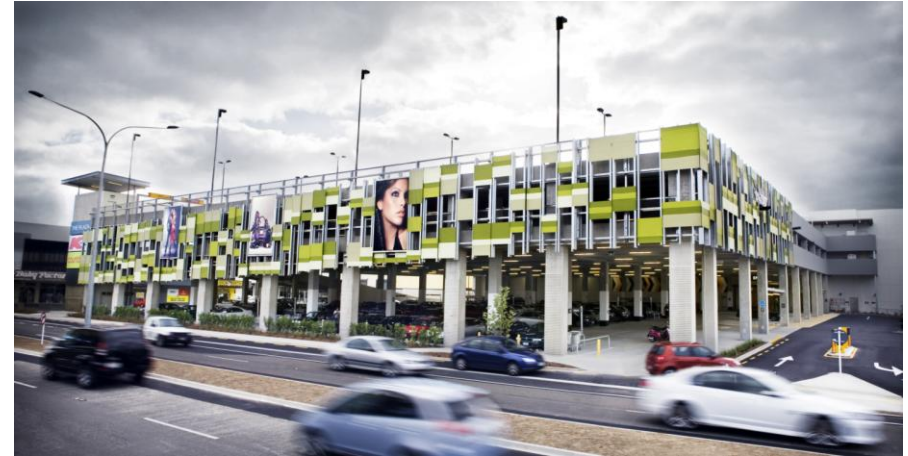
New three-level carpark viewed from Ferguson Street
