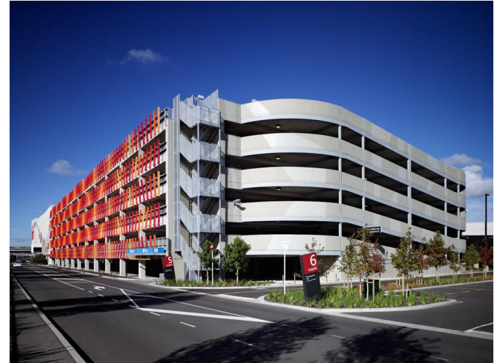
North-east multi-storey carpark
